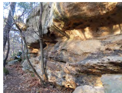
Figure 36. Formation of cavities in the Triassic sandstones (A40 Bois du Four).
